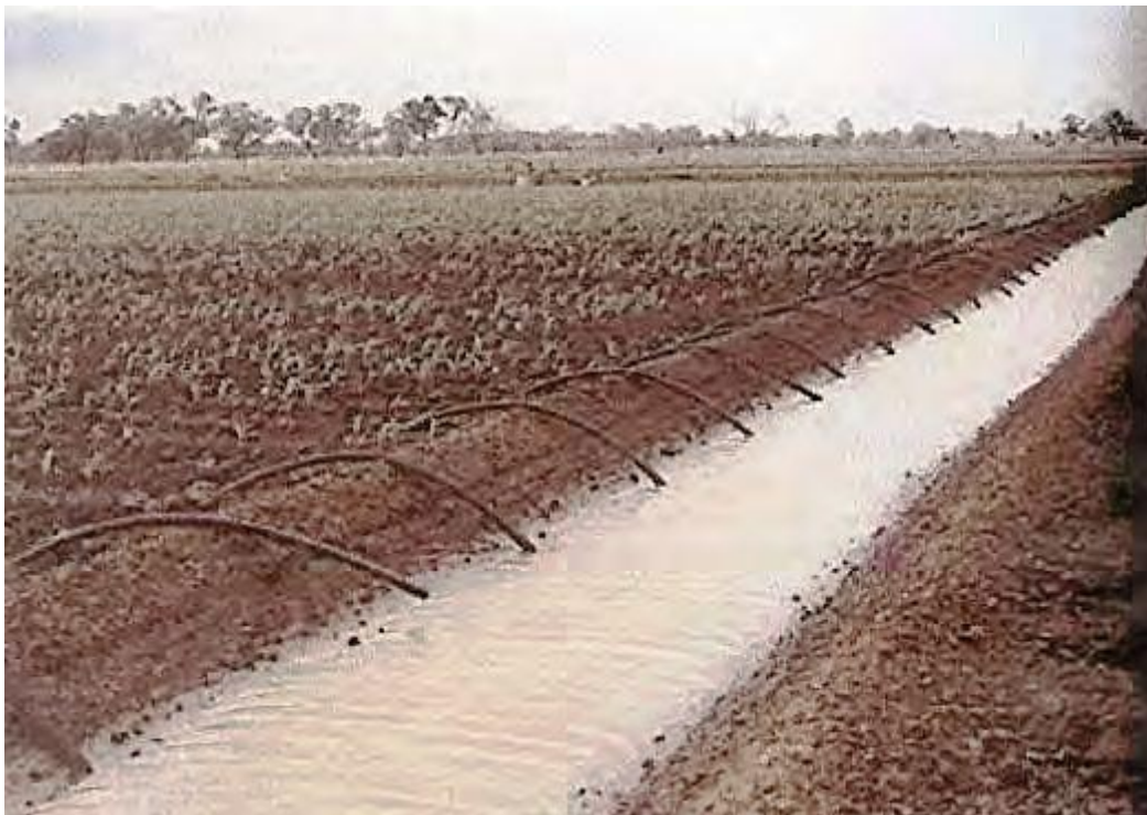
Figure 8-19: Typical Siphon tube systems in Operation
