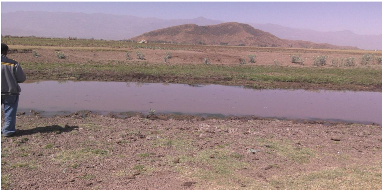
Figure 6: Diversion Point of Borkena River
