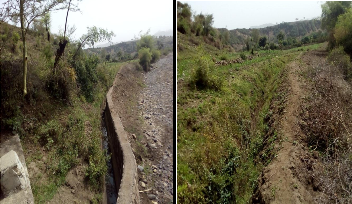
Plate 6.4: The First 0 + 900m Main Canal Route
