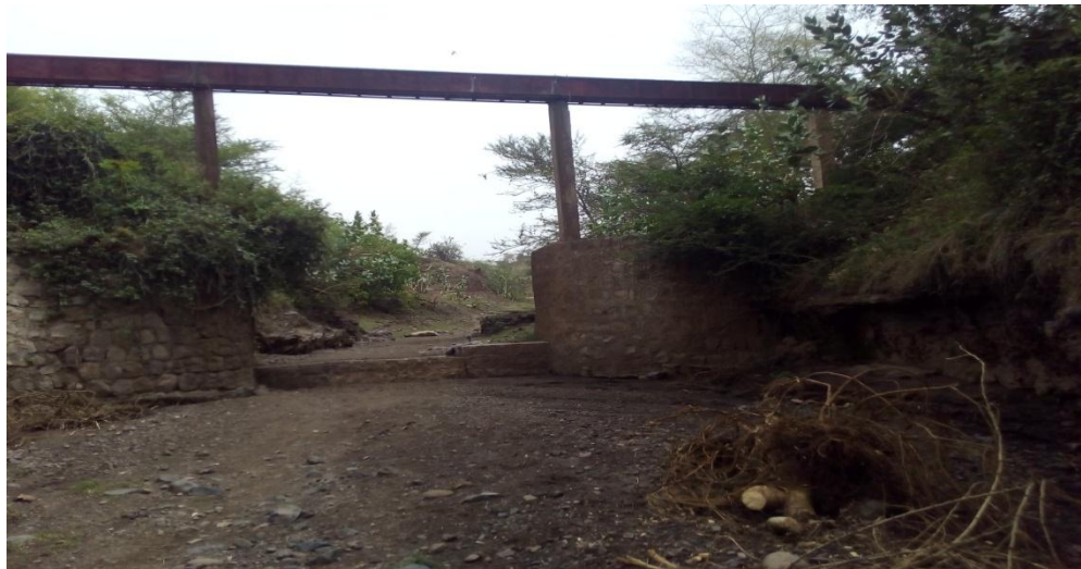
Plate 6.8: Flume at 1+400m to about 1+700m Canal Route Interval
