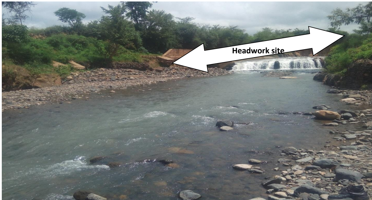
Figure 2.3 Downstream to Upstream view at headwork site
