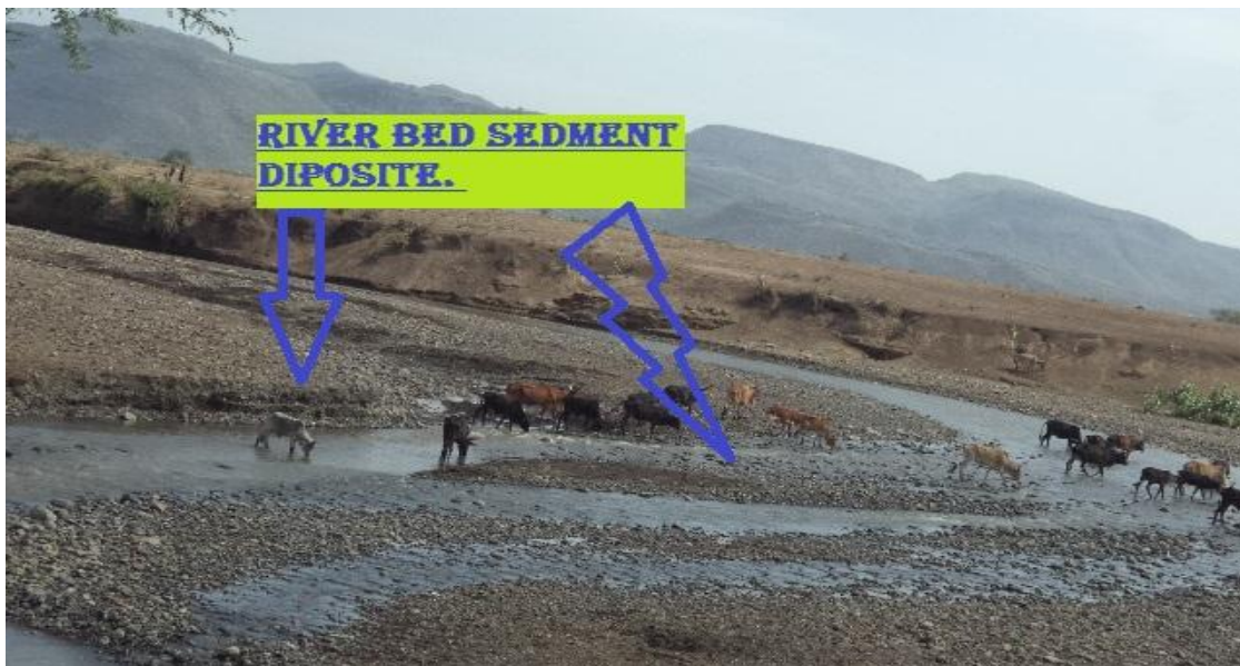
Figure 0-5: River bed at the proposed Intake site
